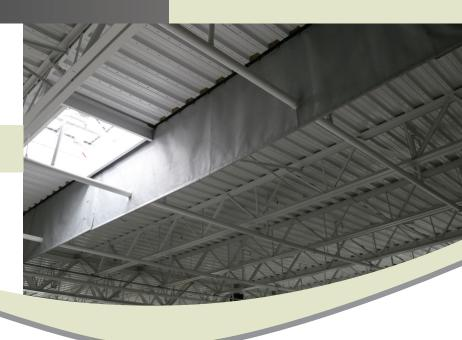
System Description. SG Draft is a cost-effective, static curtain strategy for warehouses and manufacturing environments, used in both sprinklered and nonsprinklered buildings for automatic smoke removal. Draft curtains channel the ceiling jet away from the fire and out of the building via roof vents to remove the smoke or delay sprinkler activation.
